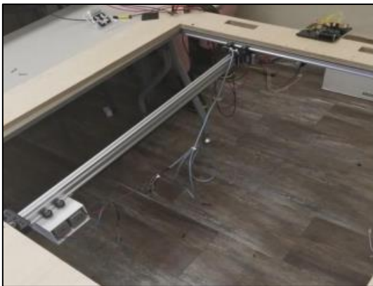
Fig.7- A shortened primary gantry arm used to test 2018 BSEN Jr. Design cable management system [3].
